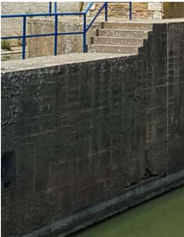
Damaged wall of the lower chamber of the canal lock pier
