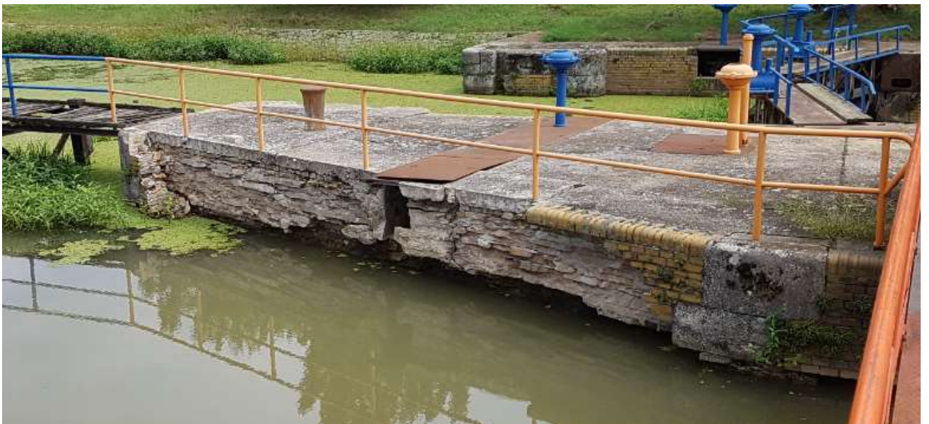
Damaged wall from the pier to the floodgate
