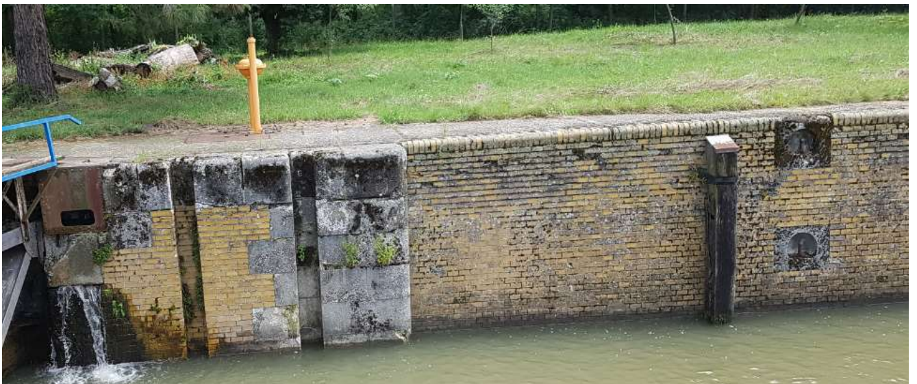
Damaged left wall of the canal lock chamber
