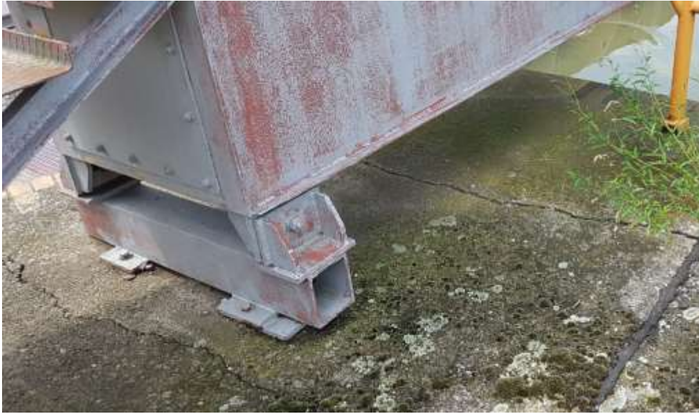
Subsidence of the left support of the pedestrian bridge on the canal lock wall - upstream view
