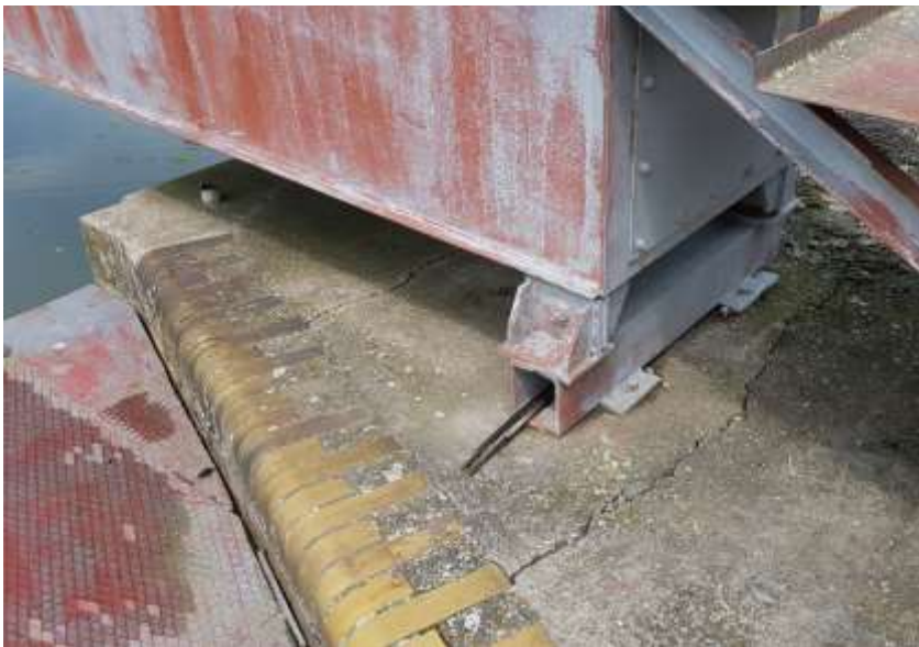
Subsidence of the left support of the pedestrian bridge on the canal lock wall - downstream view
