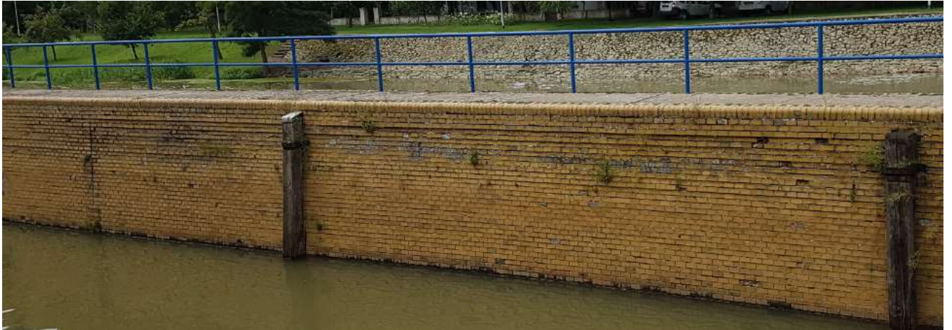
Damaged right wall of the canal lock chamber
