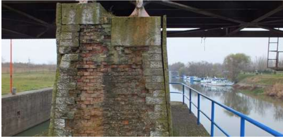
Damaged abutment
