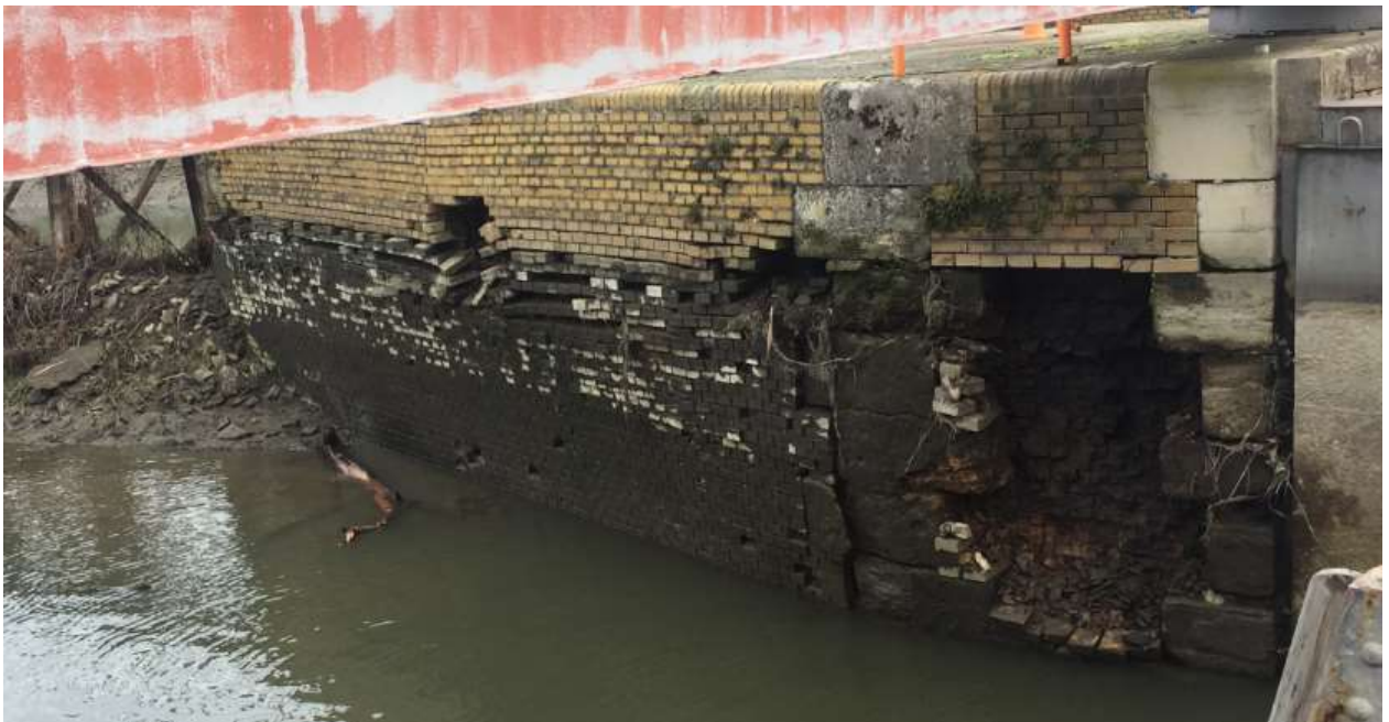
Damaged wall from the pier to the floodgate at a lower water level - close-up
