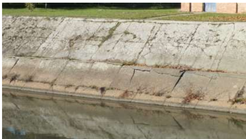
Damaged concrete lining of the canal
