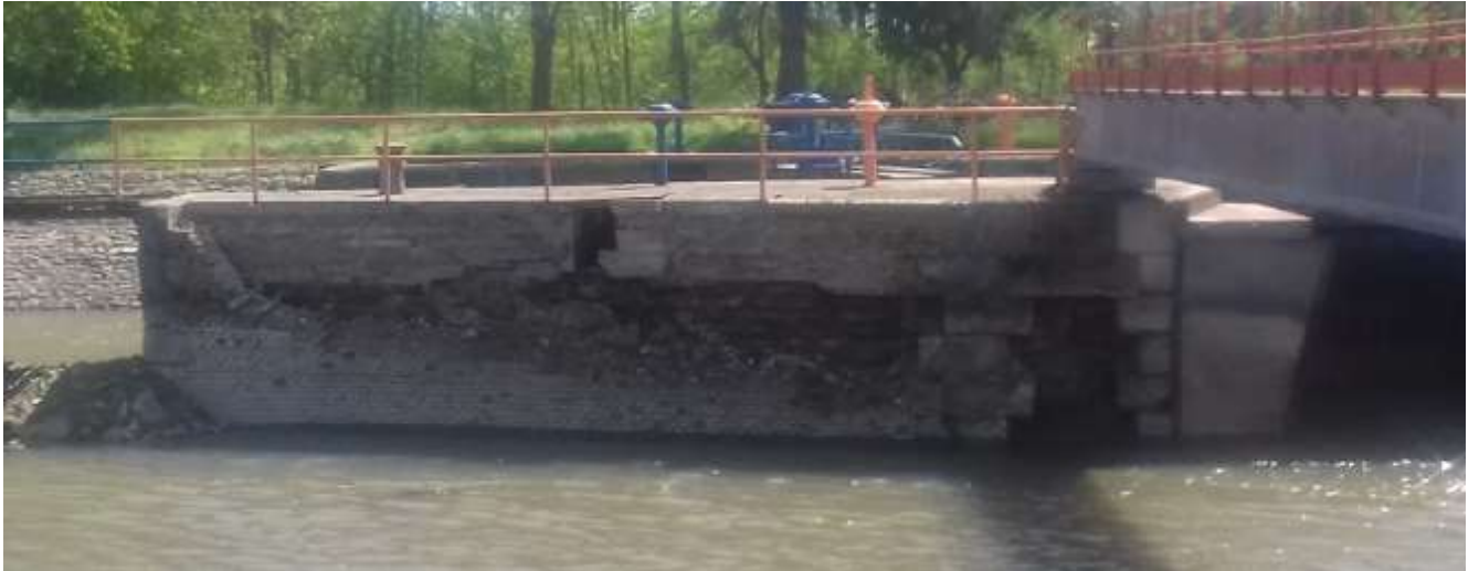
Damaged wall from the pier to the floodgate at a lower water level
