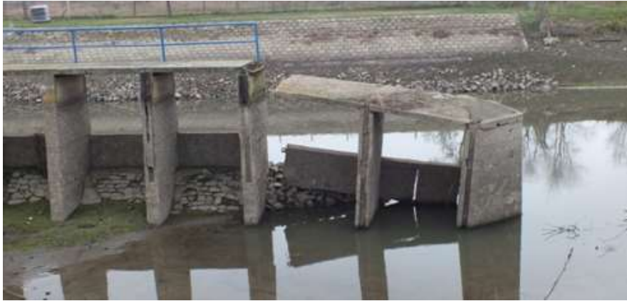
Damaged last two spans of the pier
