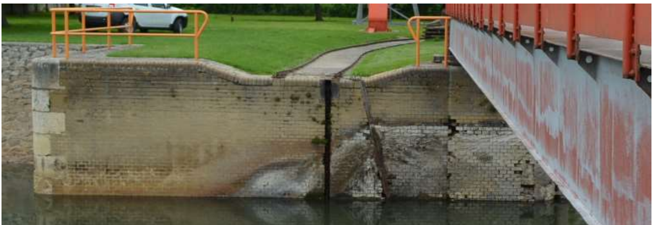
Damaged bank wall at the right bridge support
