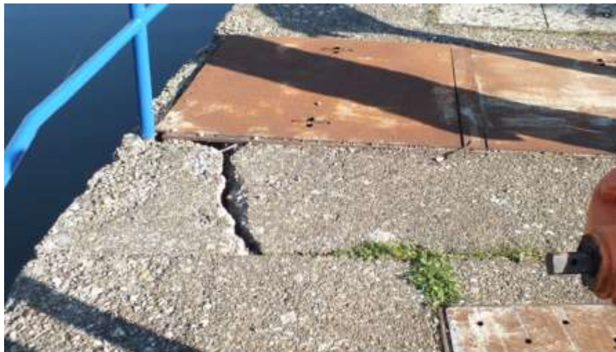
Damaged pathway on the wall of the canal lock
