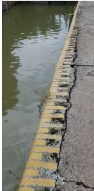
Damaged pathway on the right wall of the canal lock
