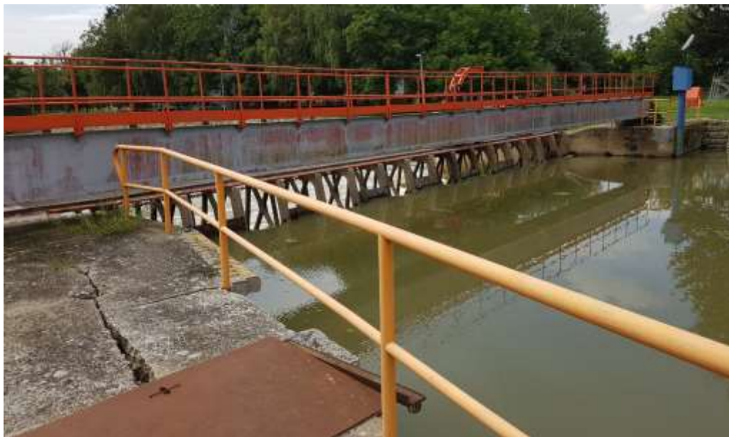
Damaged pathway on the right wall of the canal lock, in the area of the damaged wall from the pier to the floodgate
