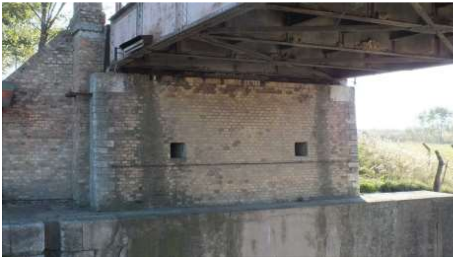
Damaged abutment
