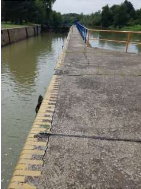
Damaged pathway on the right wall of the canal lock
